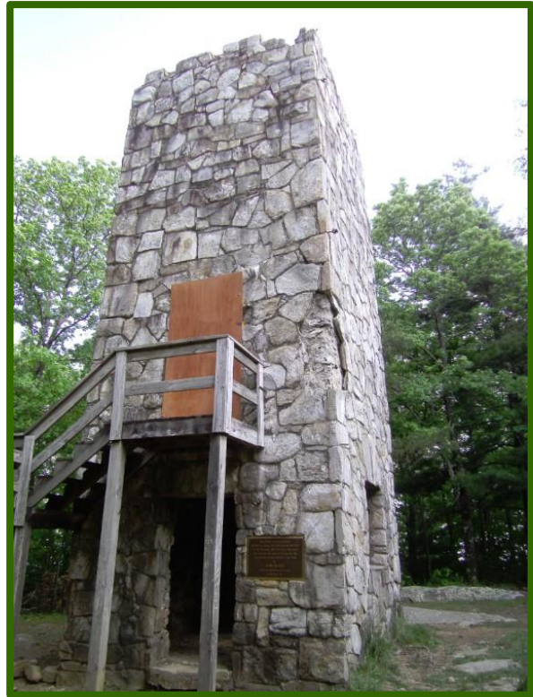
Exterior view of the front of the fire tower
