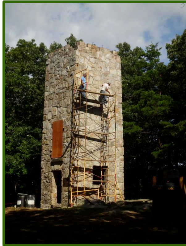
Local stone was used to replace and repair missing and damaged stones on the tower.
