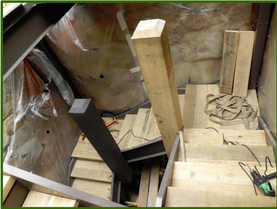
The original steps were cantilevered from the walls, but the modern steps are steel clad in wood.
